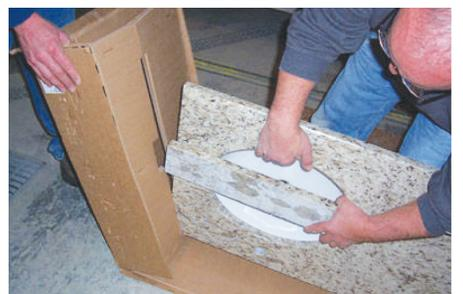
12. Slide splash out with two hands. Keep on end. **DO NOT CARRY FLAT** (to avoid breakage).
